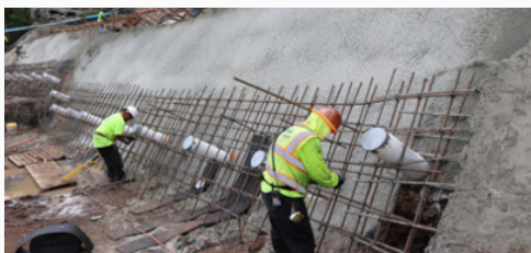
KUAHEA STREET AREA STABILIZATION PROJECT
